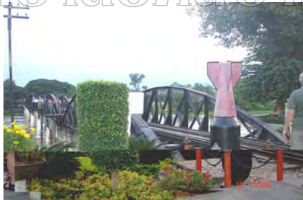
c. The bridge
